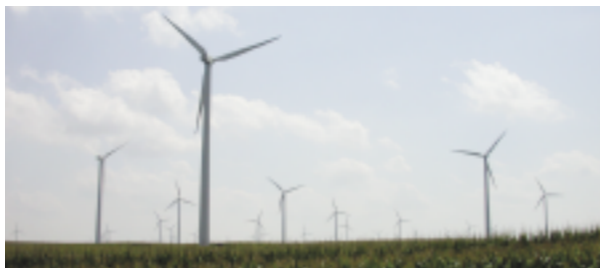
IMEA has entered into a long-term contract to purchase 70 MW of wind energy from the Lee-DeKalb wind project.
